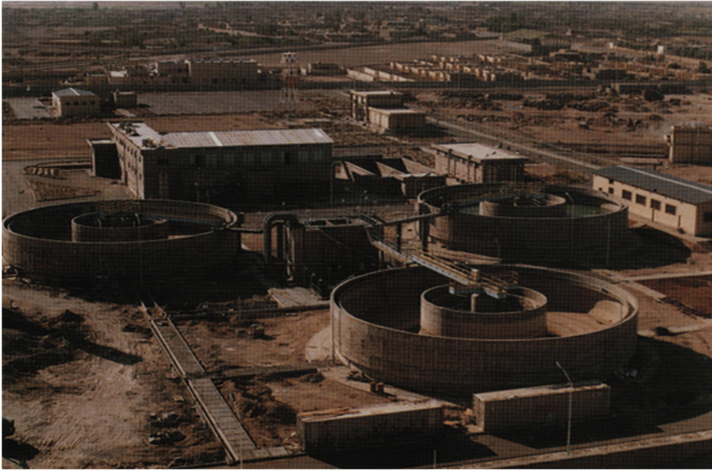
❖ Zahak Treatment Plant
