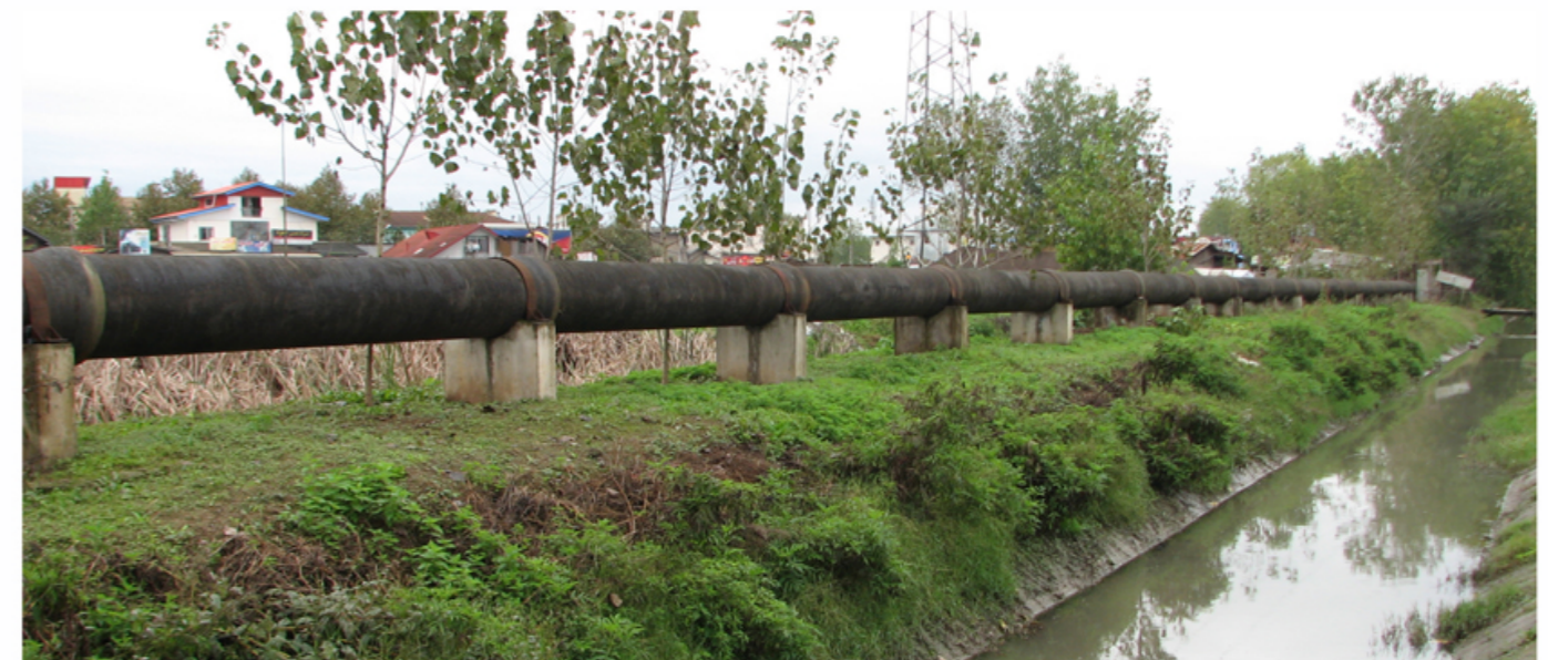
❖ A part of the water transmission line from S5 site to SW site
