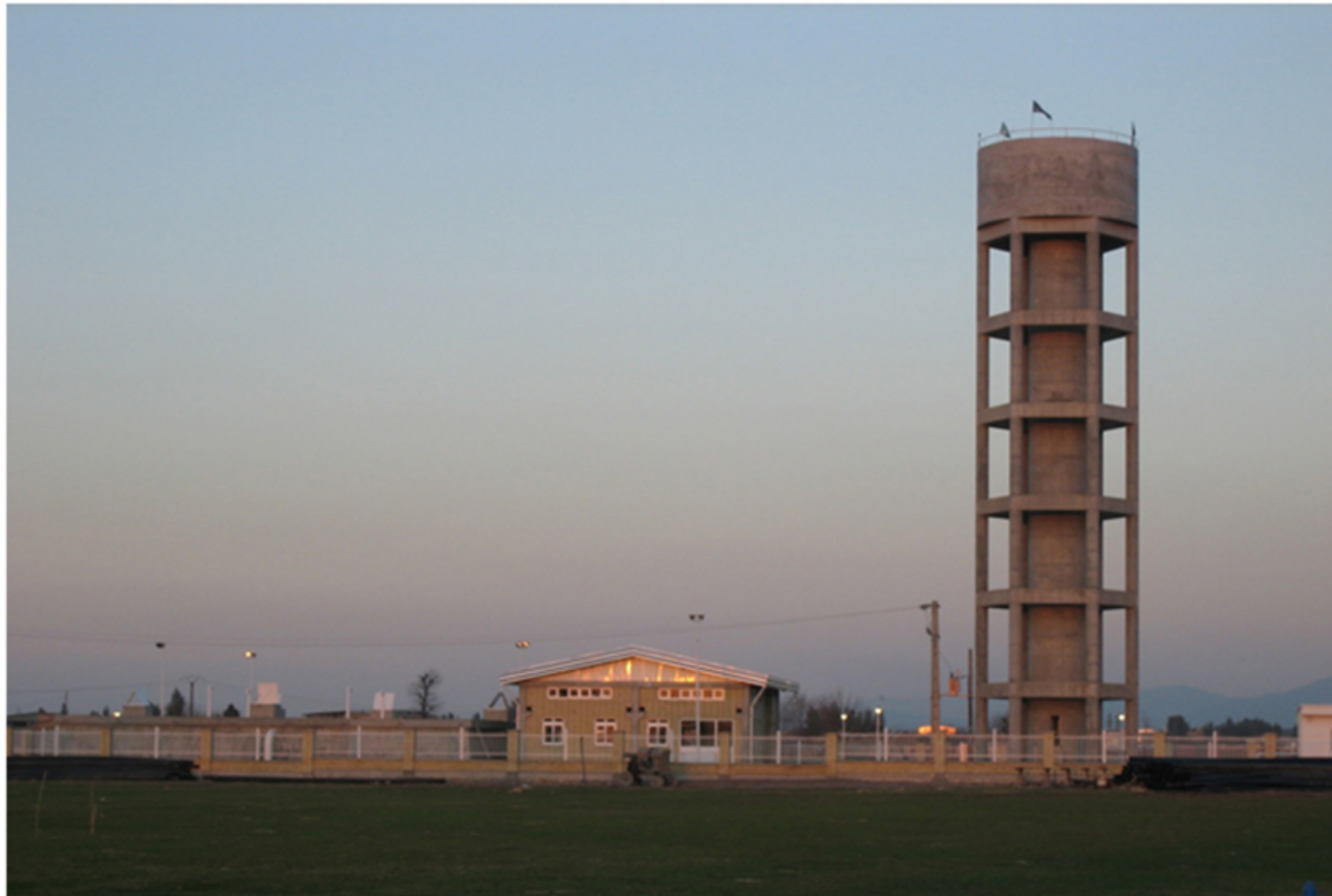
❖ Ramian 150 m 3 Concrete reservoir in Gilan Province
