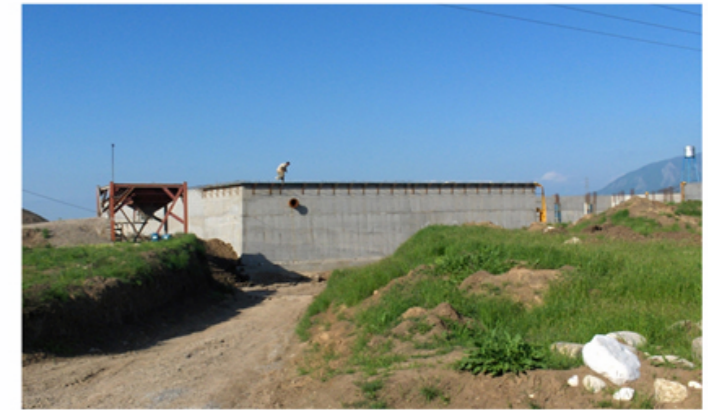
❖ Fajr 10000 m 3 concrete Ground reservoir in Minoodasht
